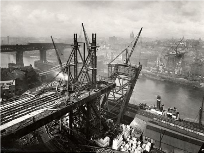
Dorman Long Collection - Building the Tyne Bridge, 1927, Courtesy of AmberSide Collection
